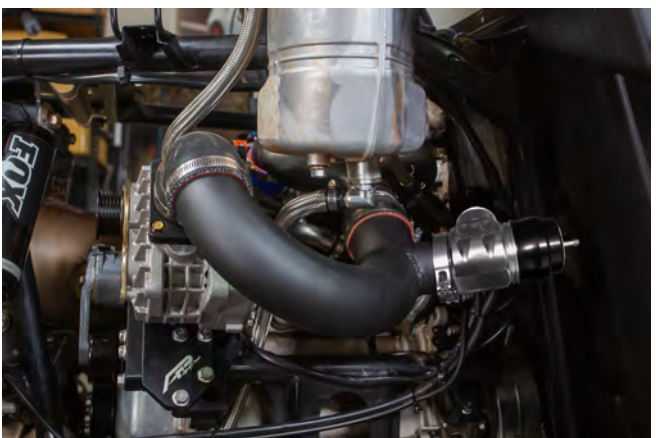
70. Install charge pipe to the supercharger outlet and trident manifold. Use the supplied 8x10mm stainless steel bolt to attach the charge pipe support bracket to the existing mounting tab located below the supercharger outlet.
